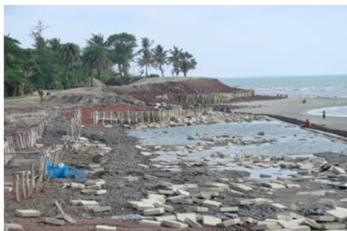
Fig. - 1. Coastal erosion in Sagar Island
